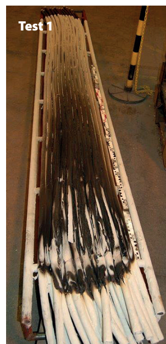
Limited damage to cables after test
